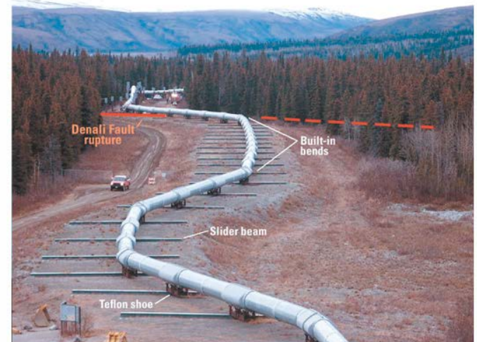
Trans-Alaska Pipeline at the Denali Fault showing major design features. Fault movement and intense ground shaking were accommodated by zigzagging the pipeline and leaving it free to slide.
