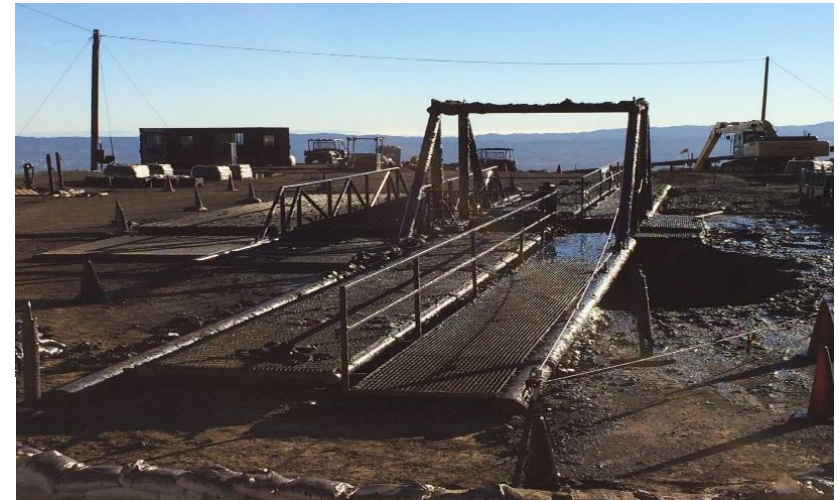
Bridge across vent to secure well head with mist abatement
